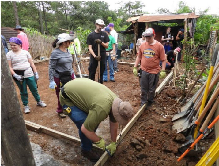
Building forms for the concrete
