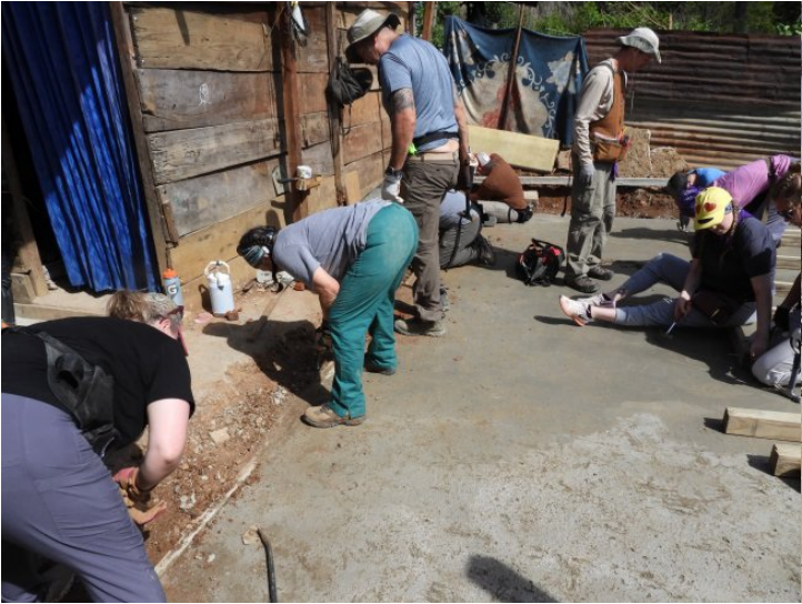
Removing concrete forms
